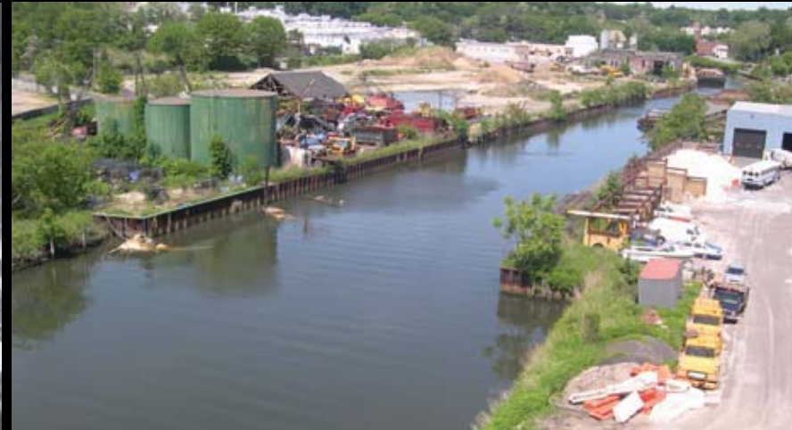
Glen Cove Creek May 2005
